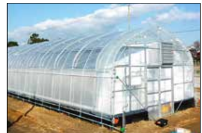
A greenhouse with a high-insulation curtain and reinforced by doubling the arched steel pipes for protection against strong winds and heavy snow
