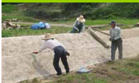
The Zoysiagrass Net-planting Technique (ZNET) facilitates the development of lawn levee banks.
