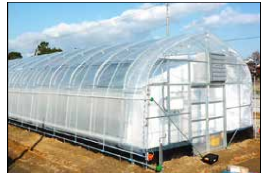
A greenhouse with a high-insulation curtain and reinforced by doubling the arched steel pipes for protection against strong winds and heavy snow
