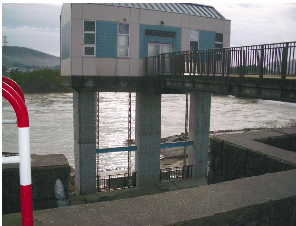
Fig.5 小千谷頭首工取水ゲート門柱 (04.10) Piers of intake gates in Ojiya Headwork
