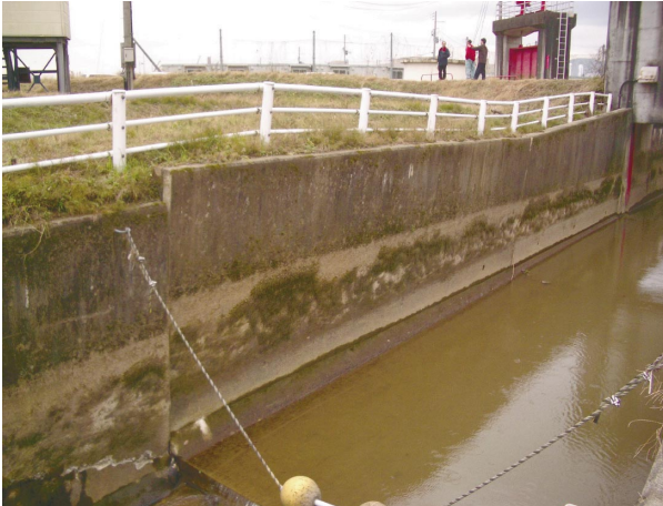
Fig.15 千谷放流工付近用水路変形 (04.10) Displacing of the main canal near the wasteway
