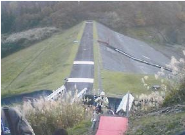
Photo 1 川西ダム全景 Overall view of Kawanishi dam
